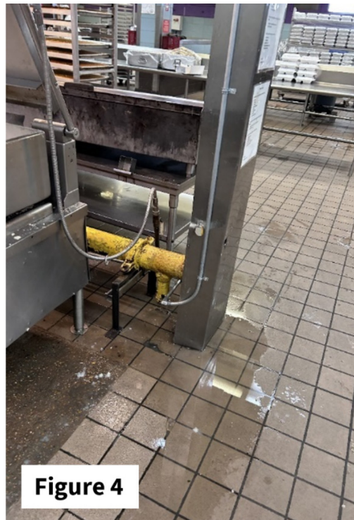
Figures 3 and 4. Leaking Vent (left), Pool of Liquid Directly Under the Leaking Vent (right), Observed March 4, 2025
