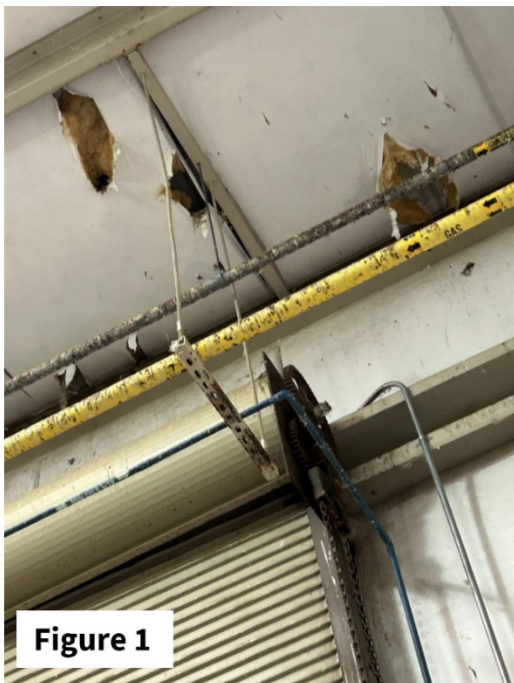
Figures 1 and 2. Deteriorated Ceiling in the Intake Building, Observed March 4, 2025
